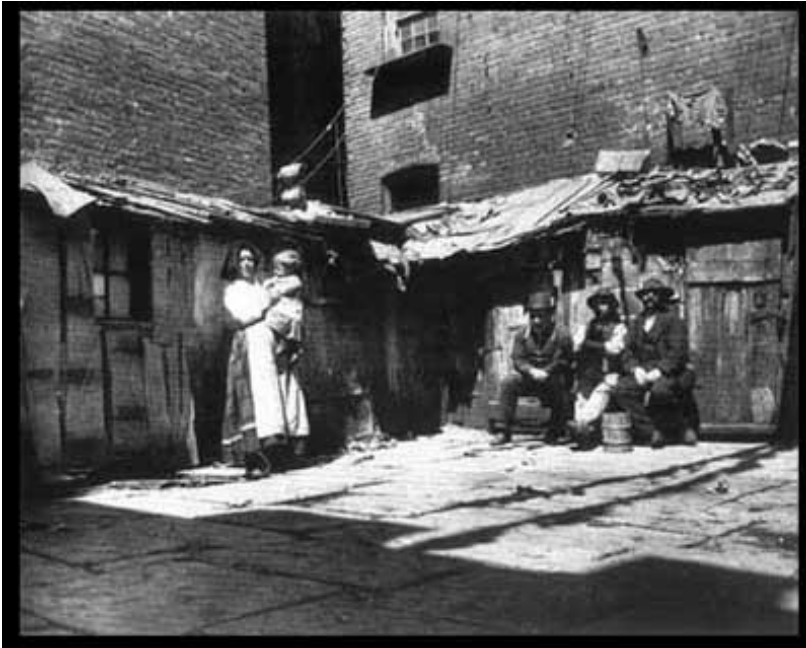
It cost a dollar a week to live in these sheds.
