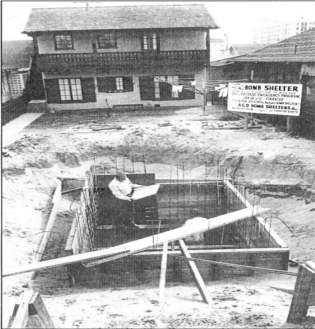
Building a Bomb Shelter
